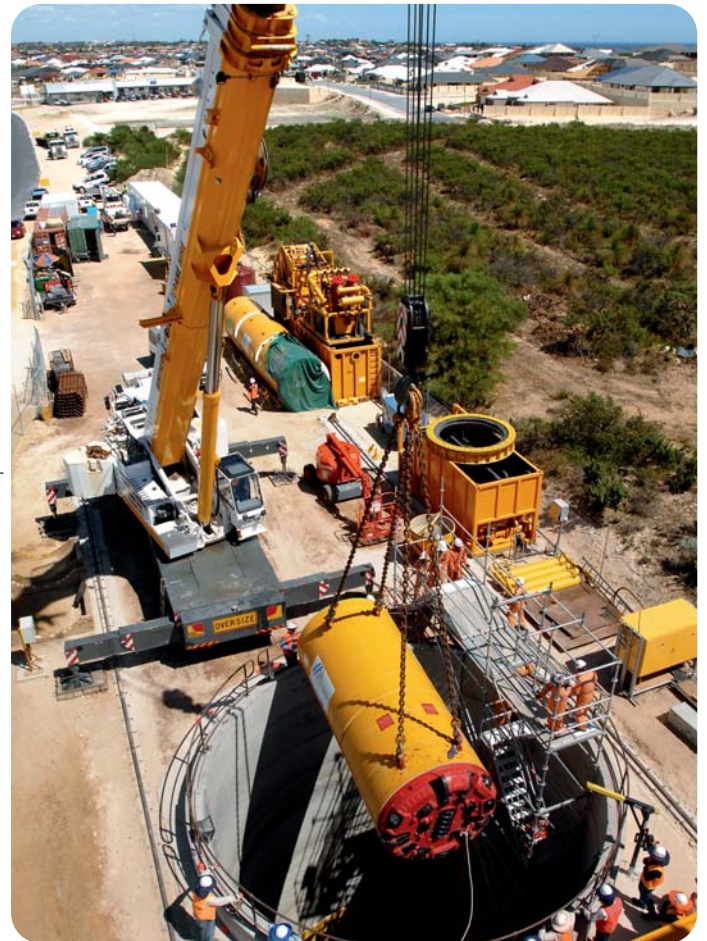
The impressive boring head is brought into position.
