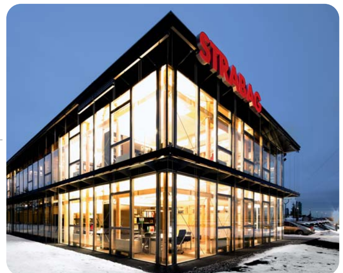
Individual construction with system – so done at STRABAG Hausleiten!
