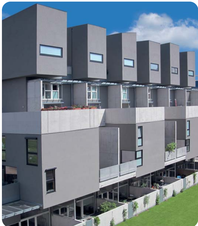
The storeys are stacked on top of and at angles to each other.
