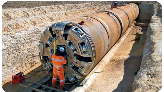
Because of the soil conditions, a dual mode TBM was used.
