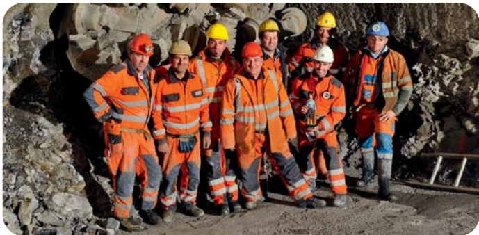
We are proud of the 50 th inclined tunnel in company history ...
