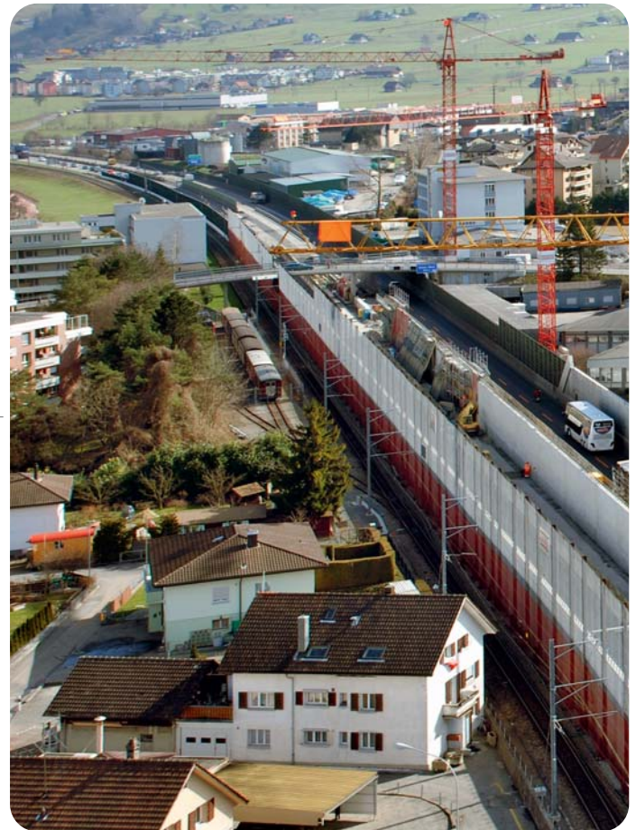
The new noise protection gallery brings quiet to Stansstad.
